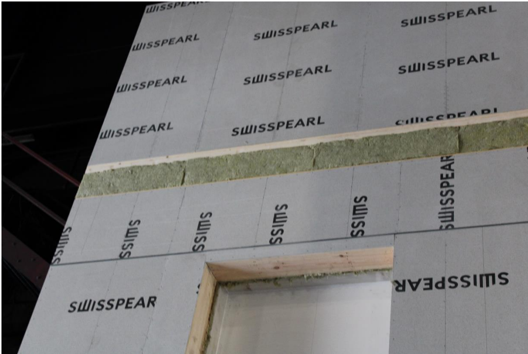
Photo No. 3 Insulation mounted between the prefabricated cassettes.
