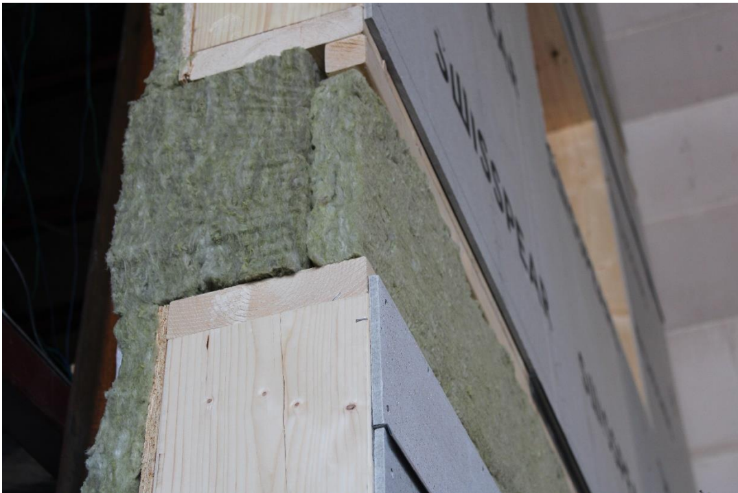
Photo No. 4 Connection between prefabricated cassettes.
