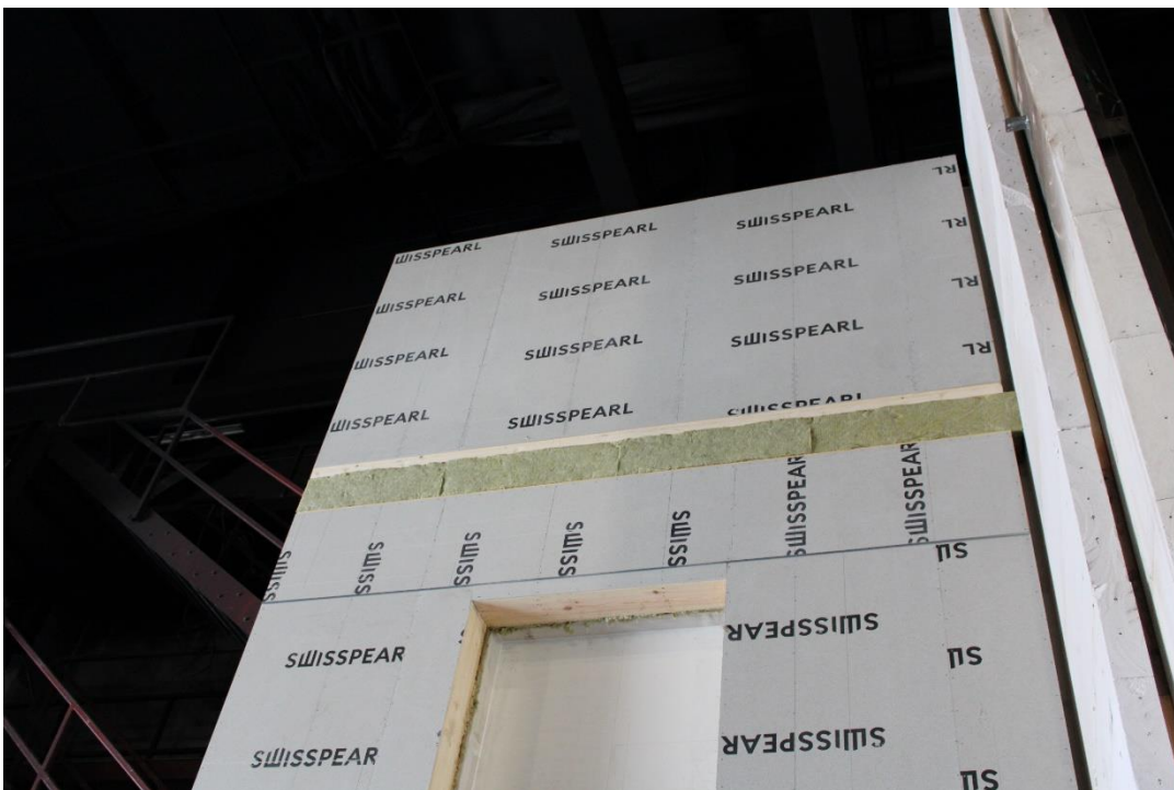
Photo No. 2 Fixing of prefabricated cassettes.
