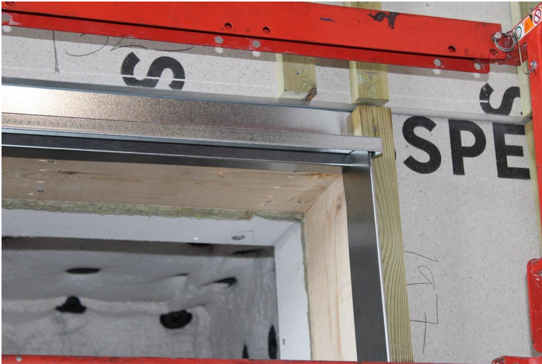
Photo No. 5 Steel flashing around window mounted.
