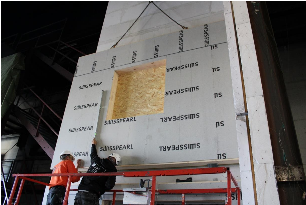
Photo No. 1 Prefabricated cassettes being mounted.
